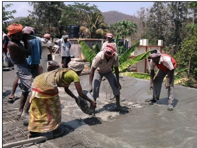
Workers building the roof on the presbytery addition
