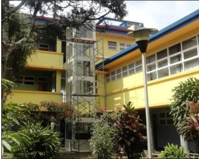
The newly installed elevator at the school
